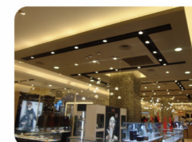
商业场所泛光照明 Market floodlight lighting
